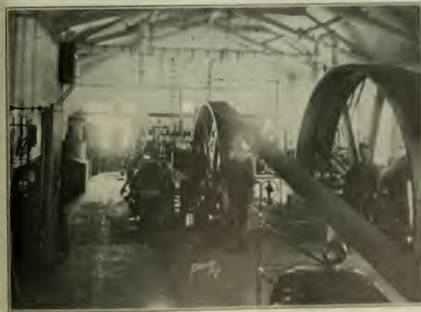
TWO VIEWS IN THE ENGINE ROOM OF THE MUNICIPAL PLANT AT WARREN, N.Y.
